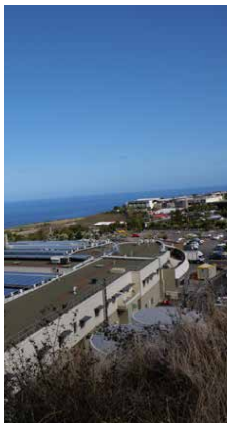
Centre commercial - Portail - Saint-Leu
